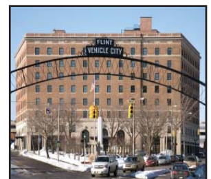
Image courtesy of Kraemer Group
