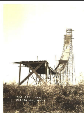
Ski Jump under construction.
